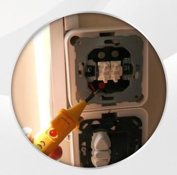
Always remeber to turn off power supply before installing any module!
