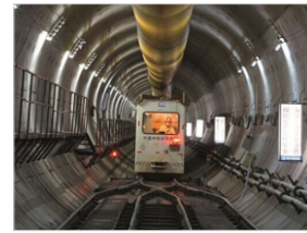
Shenzhen Metro Line 20 Project
