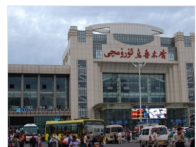
Urumqi Train Station Optical Fiber Communication Project
